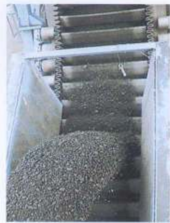
Shiploading, coal, 3,000 t/h
