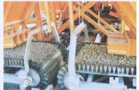
Concrete mixing plant, sand and gravel, 200 t/h
