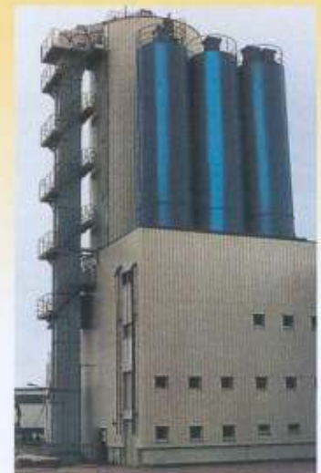
Silo feeding, sand and gravel, 250 t/h
